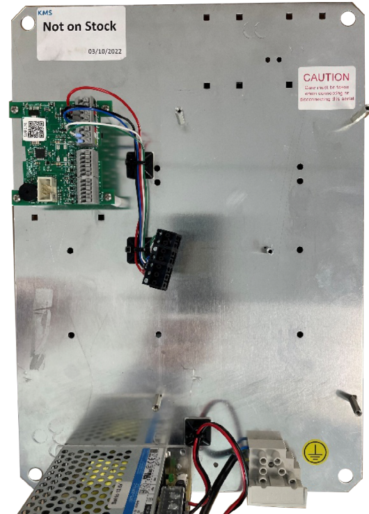
FIGURE 9.3B OLD SYSTEM CONTROLLER REMOVED
